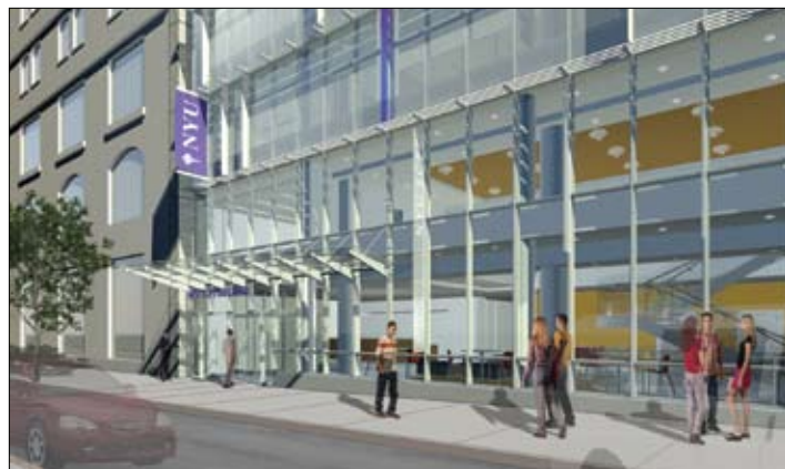
New façade, 7 East 12th Street.
